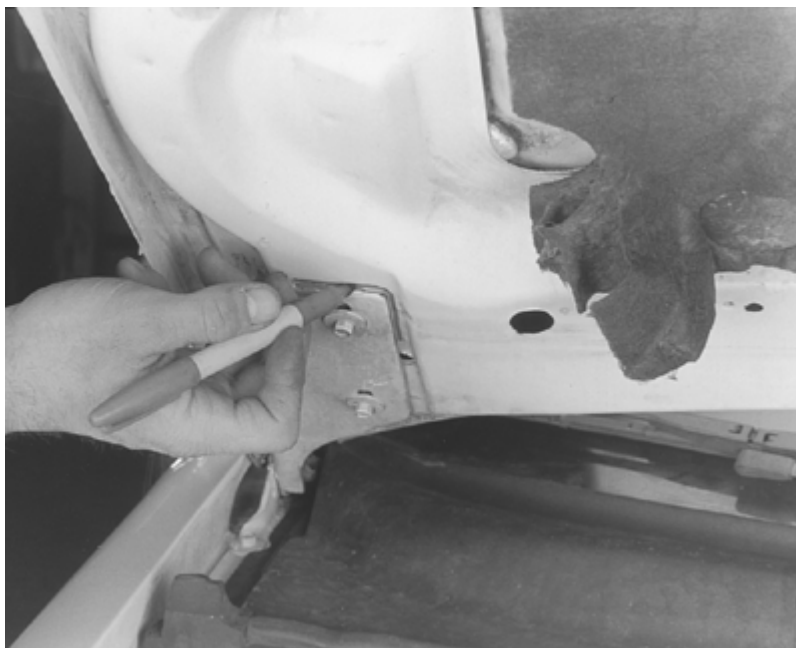
Scribe the hood hinge locations on the hood for installation purposes
